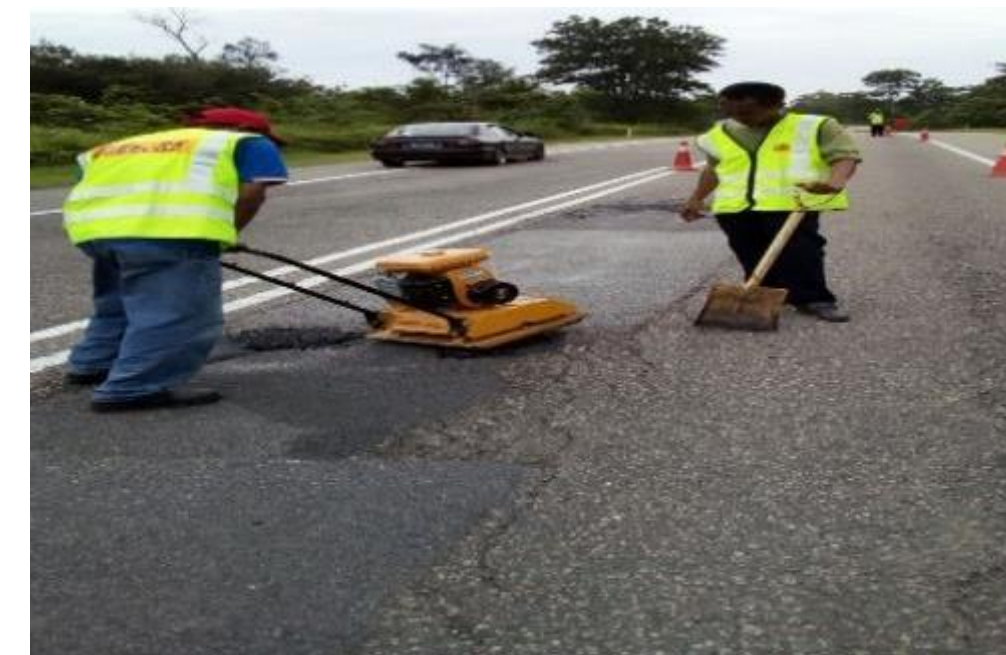
Patching of potholes
