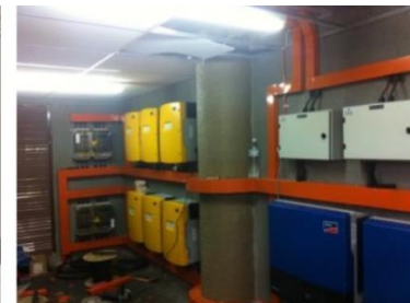
Inverter and battery installation
